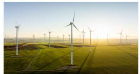
Wind turbines & wind farms
